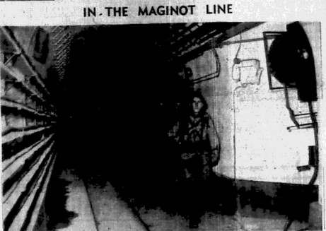
French soldiers are seen marching along an underground passage in the Maginot Line. The picture shows the complicated electrical and telephonic wiring, and the narrow gauge railway line, for electric trains, will also be observed.
