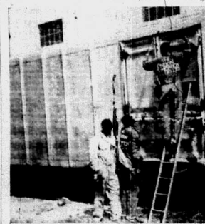
Operators working the hours of a railway track in preparation for the new railway line East Africa by the London-Funguon Company (Kenya) Limited.
