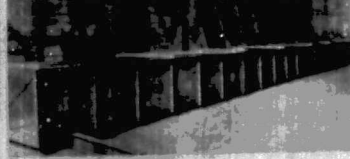
4'0" x 2'0" x 30 feet Beam Assembled.
