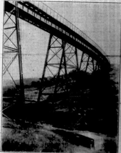
One of the steel truss bridges on the Kenya and Uganda Railway.
