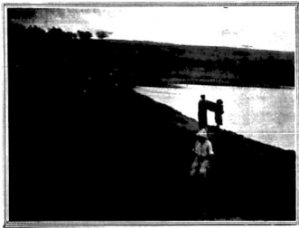
On top of the dam
