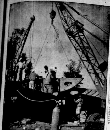
A partial view of the ship is lifted into position during the reconstruction of the R.M.S. Victoria at Scotland. Glasgow, will be ready for service again on Lake Victoria by the middle of this year.
