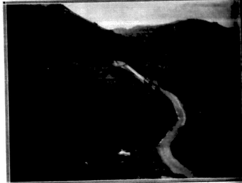
Part of the new road from Kabale in the Kigezi District of Uganda to the Congo. The road is a fine piece of engineering and passes through magnificent scenery. Picture: Miss E. Paine.
