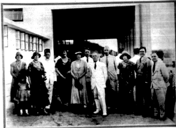
Mrs. Field Jones after opening the new bath.
