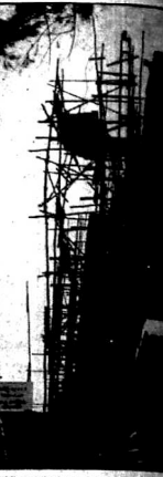
Scaffolding at the front of the new Post Office.
