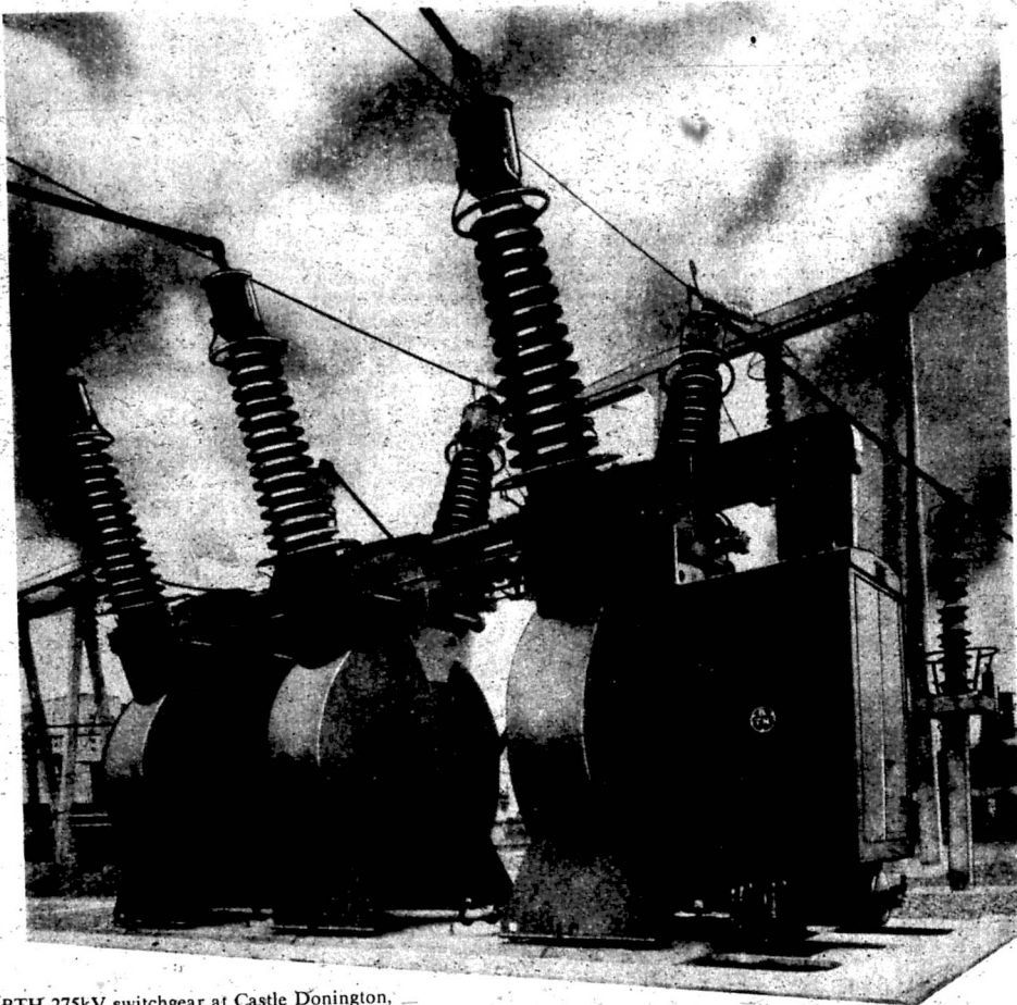
BTH 275kV switchgear at Castle Donington, C.E.A. East Midlands Division.
