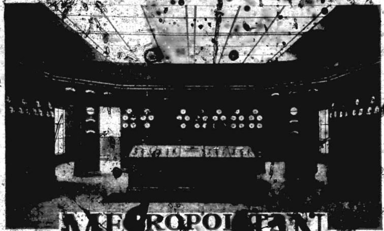
The Control Room at a large Generating Station, showing the panels and generator control desk. The panels control the "Melbo-vick" 6,000 volt triplicate bus Metalclad Switchgear installed in this station.
