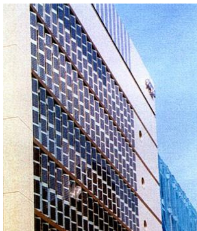
Figure 2.8: Solar Wings in an Office Building in Switzerland with Fixed BIPV Louvres [26]
