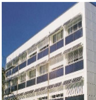
Figure 2.9: Moveable Sunshades in a Commercial Office Building in Switzerland [26]
