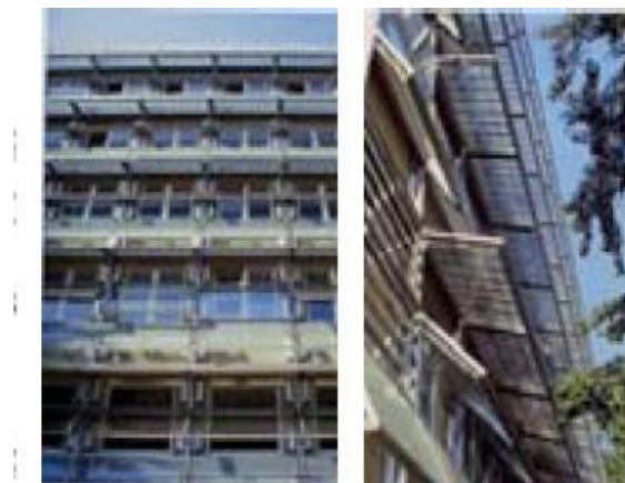
Figure 2.7: Fixed Sunshades in the SUVA Building, Switzerland Built in 1993[26]
