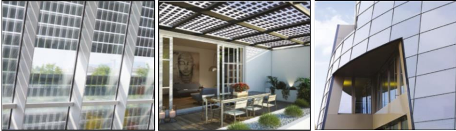
(a) PV Curtain Wall (b) Glazed Façade PV (c) Rain Screen Façade PV
