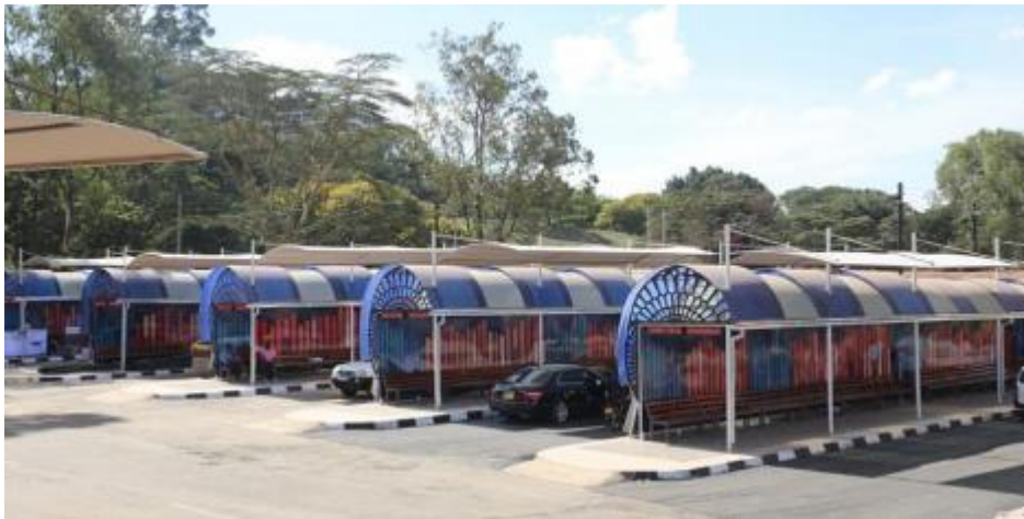
Figure 3. 4: View of the Green Park Terminus at the Old Railways Club
