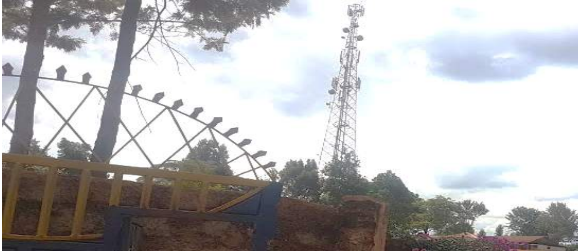
Figure 21: Communication Mast near Gachoka Primary School (Field Survey, 2019)
