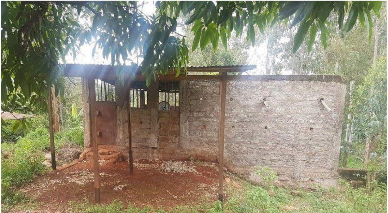
Figure 53: Coffee Collection Centre (Field Survey 2019)
