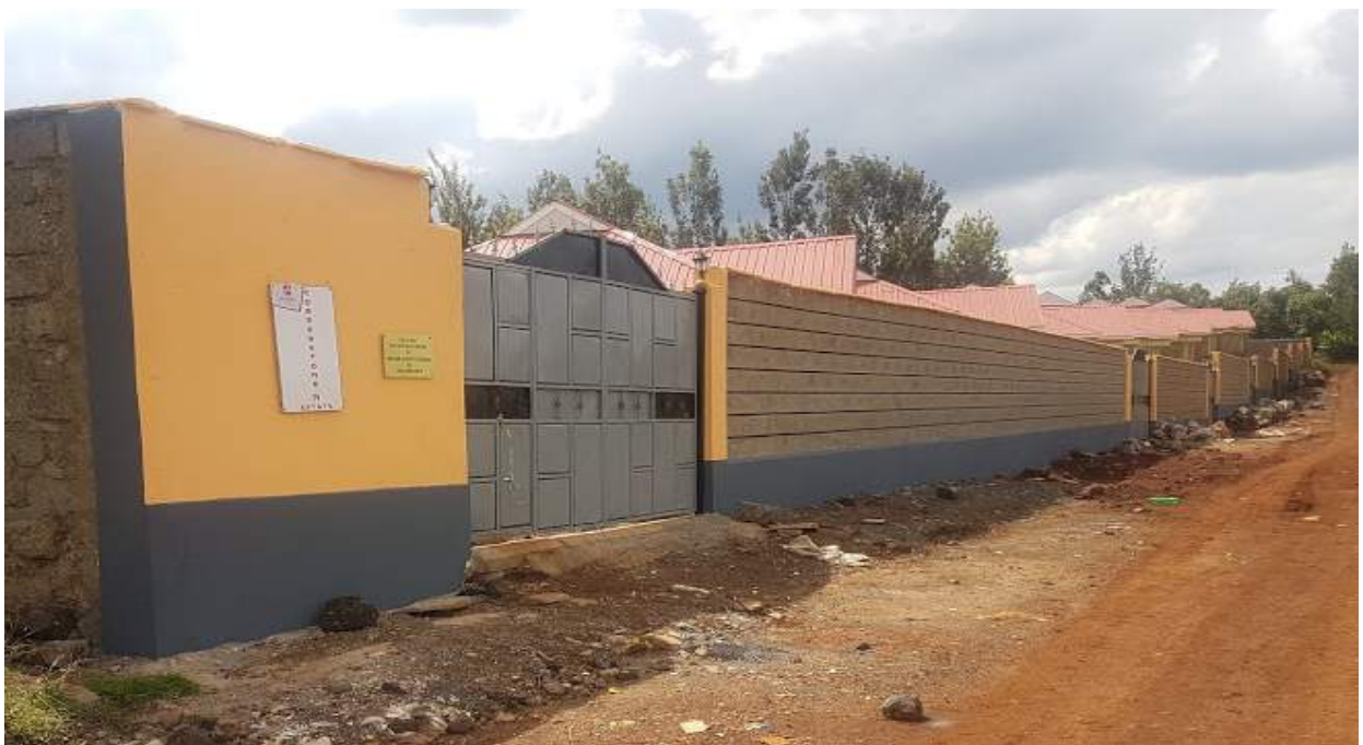
Figure 41: Cornerstone Estate (Field Survey, 2019)
