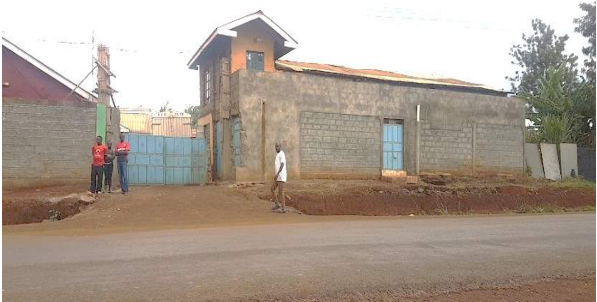
Figure 52: Steel Welding Light Industry (Field Survey, 2019)
