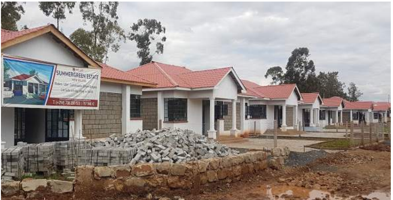
Figure 43: Summergreen Estate (Field Survey, 2019)
