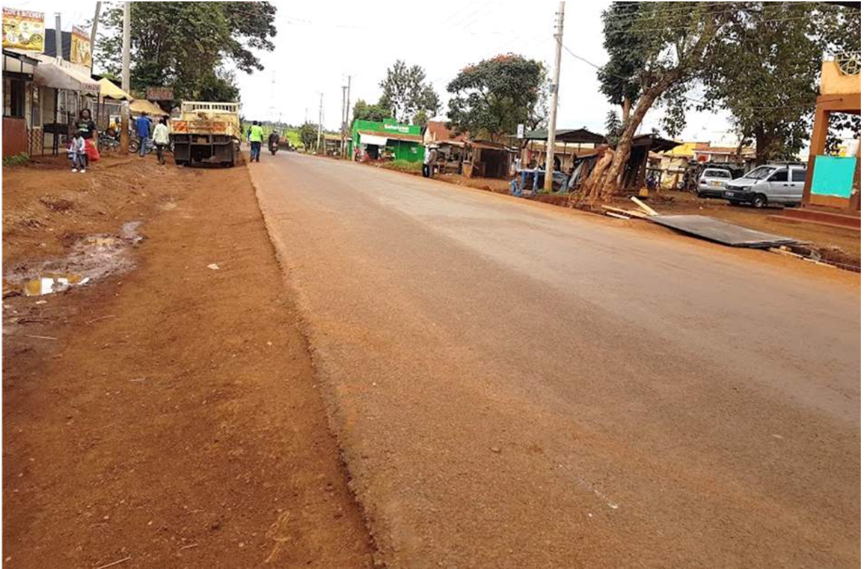
Figure 17: Kenyatta road section (Field Survey, 2019)
