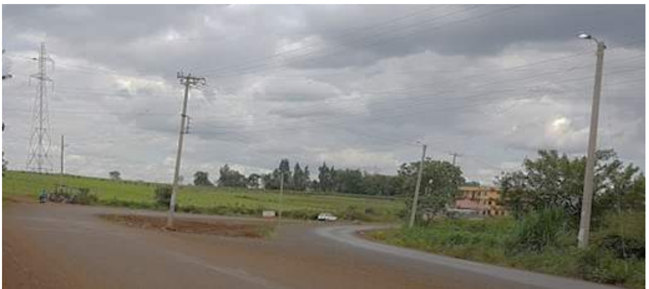
Figure 20: Illustration of Electricity Grids (Field Survey, 2019)
