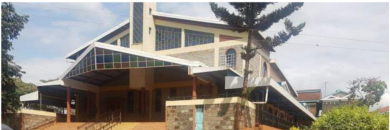
Figure 33: P.C.E.A Kimunyu (Field Survey, 2019)
