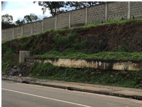
FIGURE 3 Overflowing sewer along Mbagathi link Source: Author, 2023
