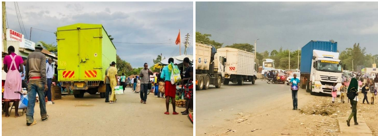
Plate 1: Roads Condition in Ahero Town
