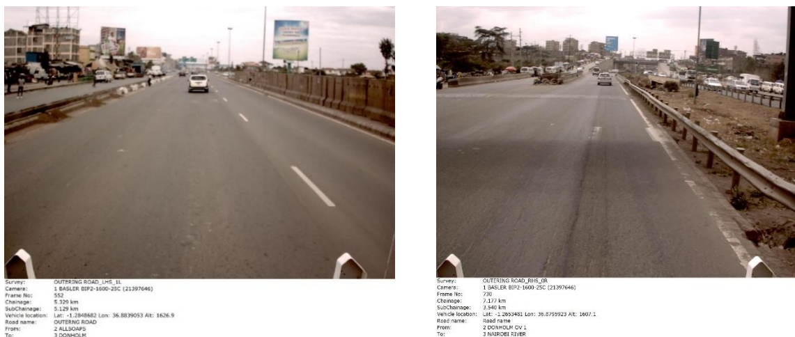
Figure 4-3: Pavement surface condition during the survey
