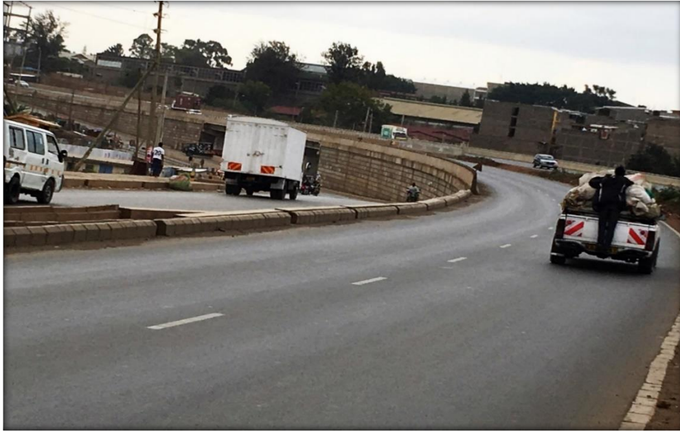
Figure 3-1: Mathari river reinforced earth section, 2021
