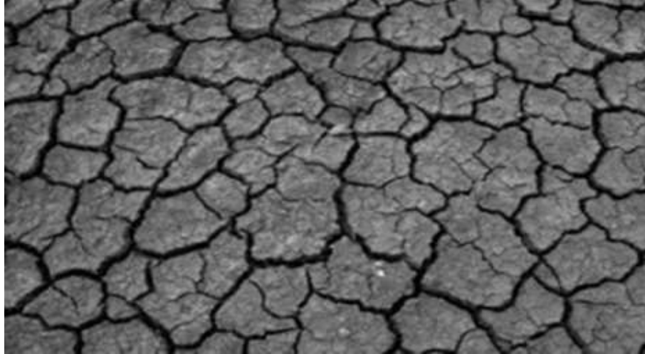
Plate 1: Black cotton soil showing heavy cracking during the dry season
