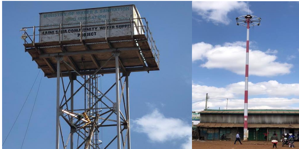
Figure 12: Community water tank and street light at Laini Saba grounds
