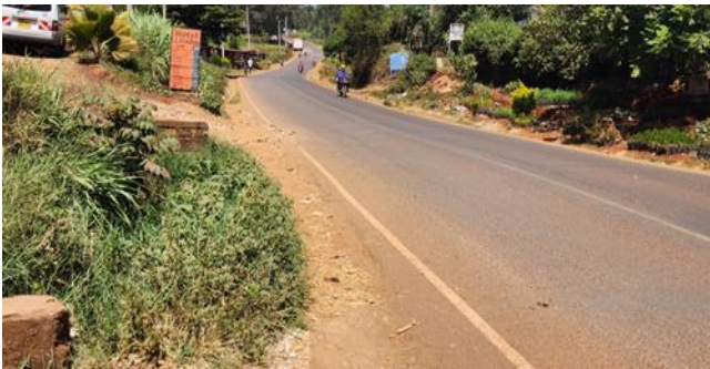
(c) Road transcends an urban setup, still in good serviceability, but in poor maintenance condition (Author, 2023).
