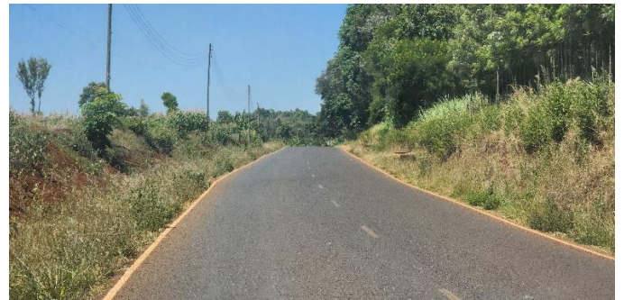
(d) Towards the end stretch of the road, a good ride quality was experienced, and the road was in good service. Poor drainage and lack of timely routine maintenance was noted (Author, 2023).
