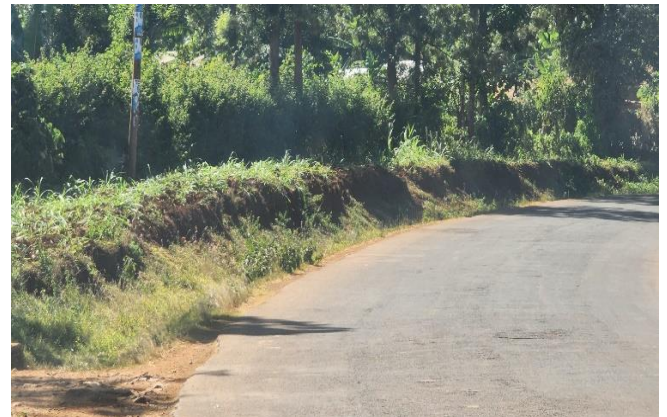
(b) Section showing the erodibility potential of the embankment slopes (Author, 2023)
