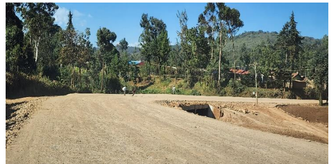
(d) Ongoing box culvert works at the road upgrading project (Author, 2023)
