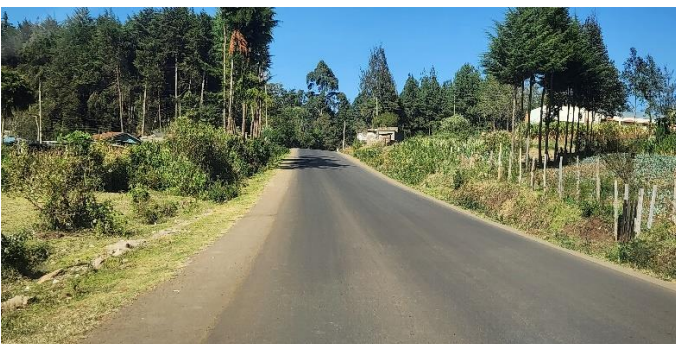
(e) Completed asphalt surfacing where upgrading works were on-going (Author, 2023)
