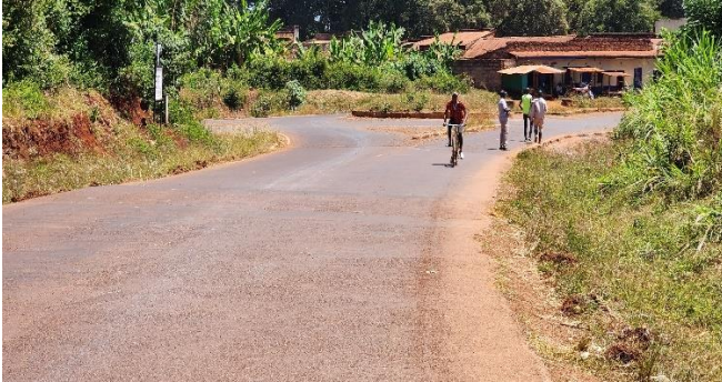
(a) Road start at Gakoigo junction. Asphalt surface intact, but poor drainage system noted (Author, 2023).
