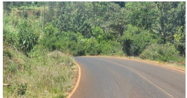
(b) Section showing the road geometry on a curve with poor visibility. Case of inadequate routine maintenance (Author, 2023).
