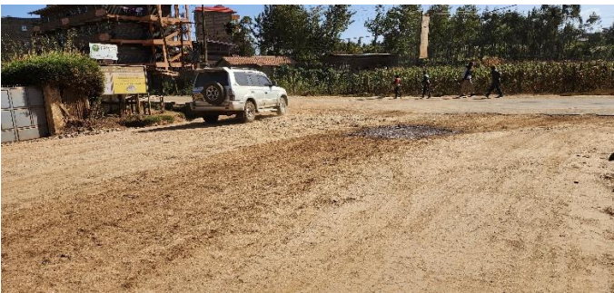
(c) Road start where upgrading works were on-going (Author, 2023)
