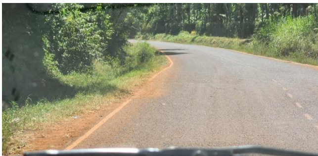
(c) Section showing a section still in good serviceability (Author, 2023).
