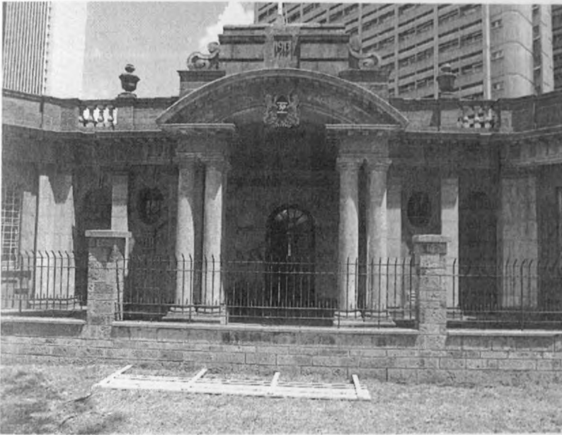
Figure 5.1: Photograph of the Old PC's Office Building.
