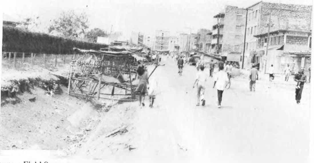
Plate 4.20: Structures Built Over Storm Water Drainage Along Northern Spin Road Making Cleaning of the Drain Difficult
