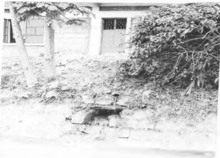
Plate 4.23: Structure Built on top of a Sewer in Dandora Area 2 (Note the raw sewer discharge into the open drain along Apudo Road)
