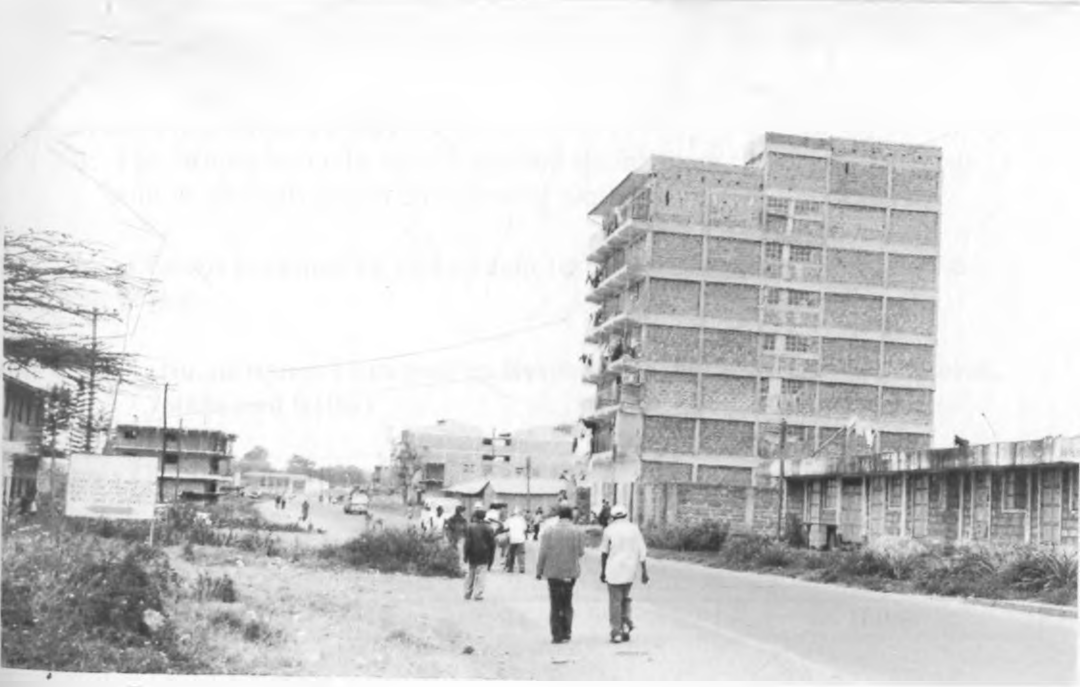
Plate 4.7 An Illegal Eight Storey Building along Komarock Road below Area 2
