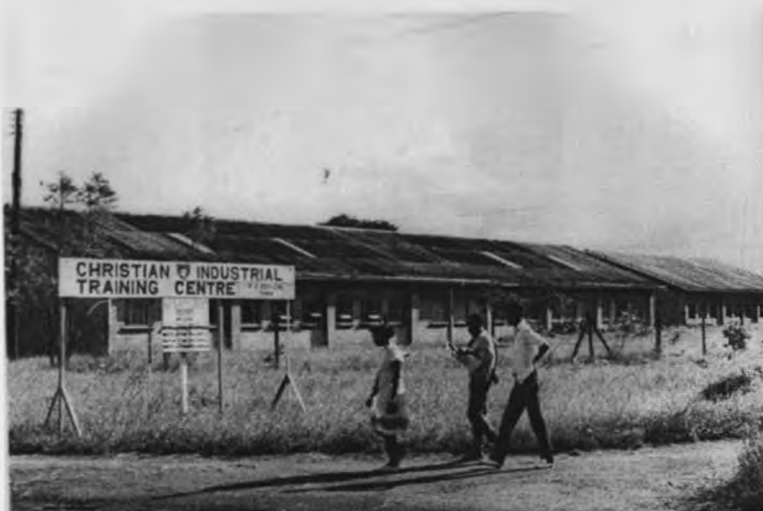
The corroded iron sheets roofing on a school building opposite KEL Chemical Factory (Daily Nation Picture)
