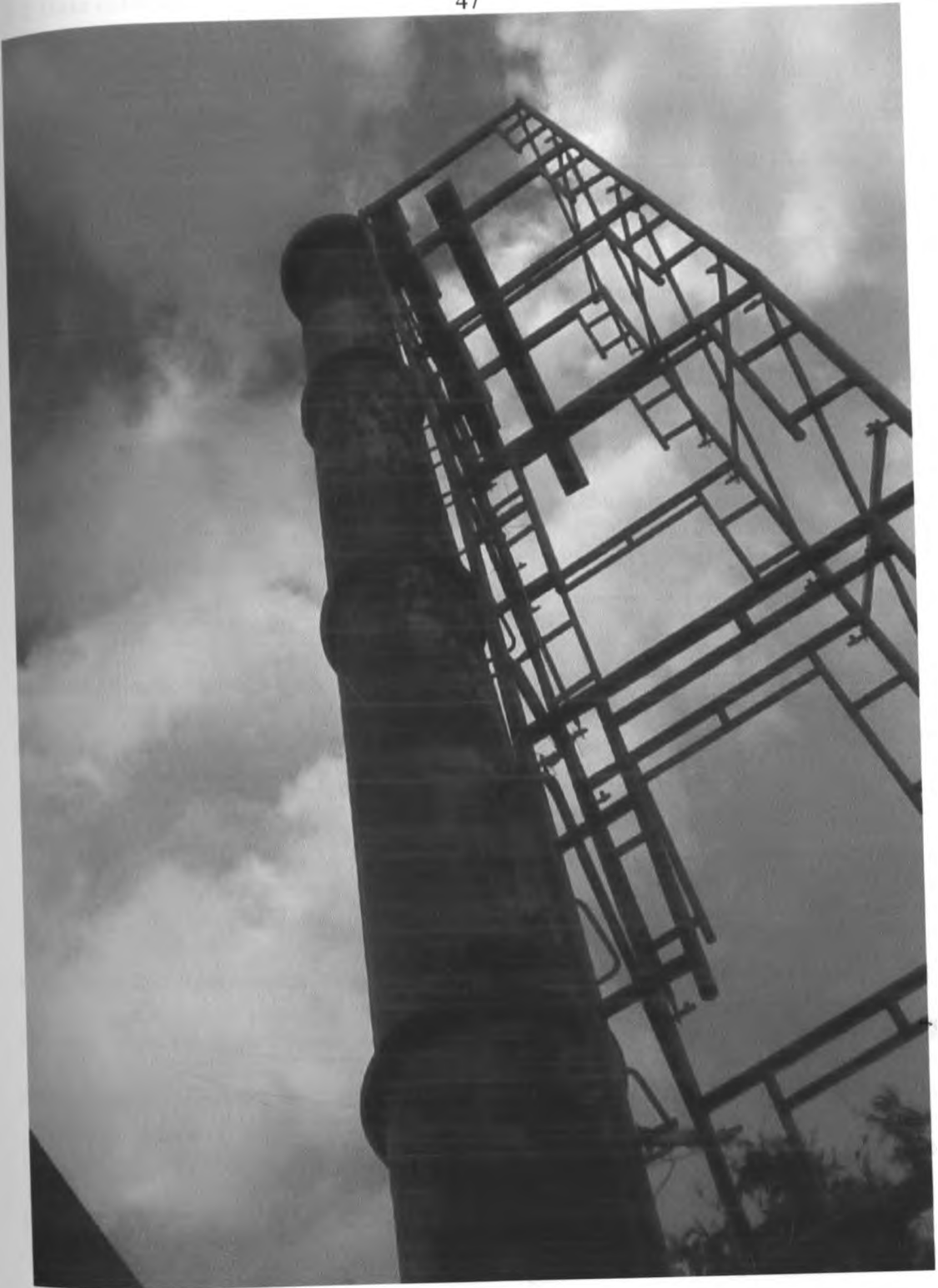
Figure 1: Standard height of an incinerators' chimney discharging fumes from study site (H3).
