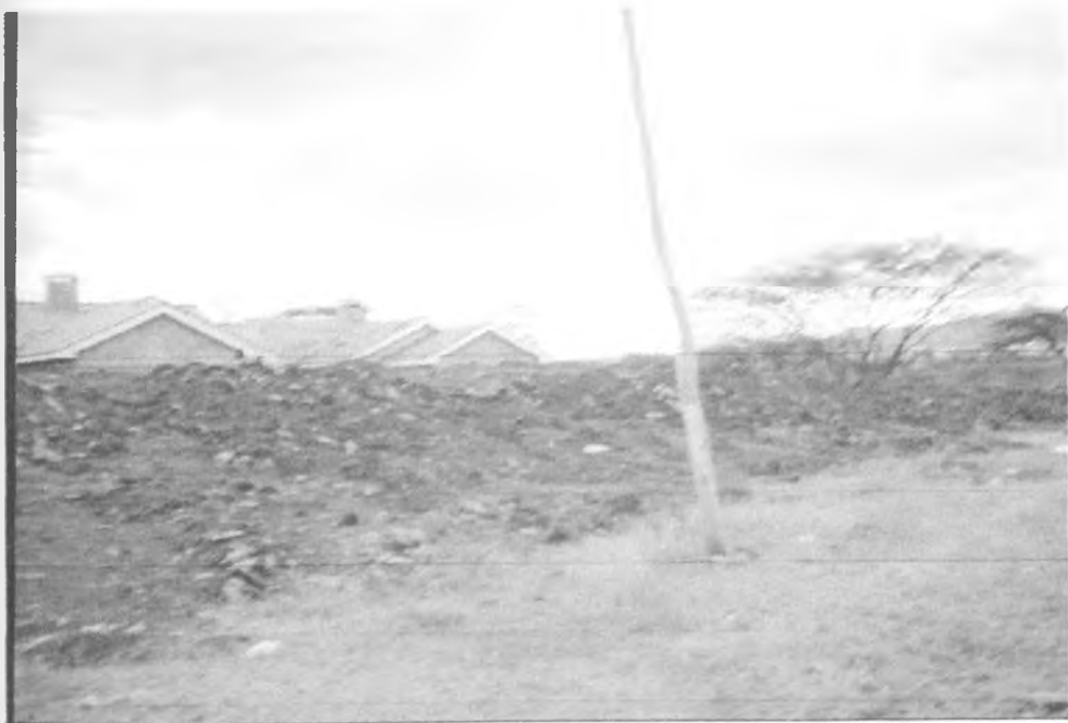
Figure 13: showing Roadside and site dumping
