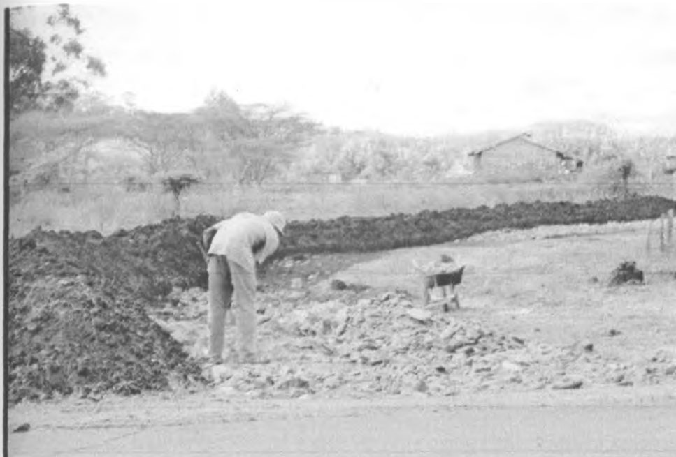
Figure 14: showing early stages of compaction and sediment generation through laying of roads
