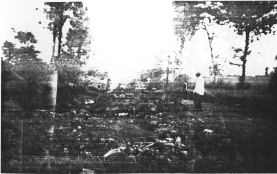
Plate 10: KTDA uses waste quarry chips to repair tea roads as observed in this photograph on Weru factory road.
