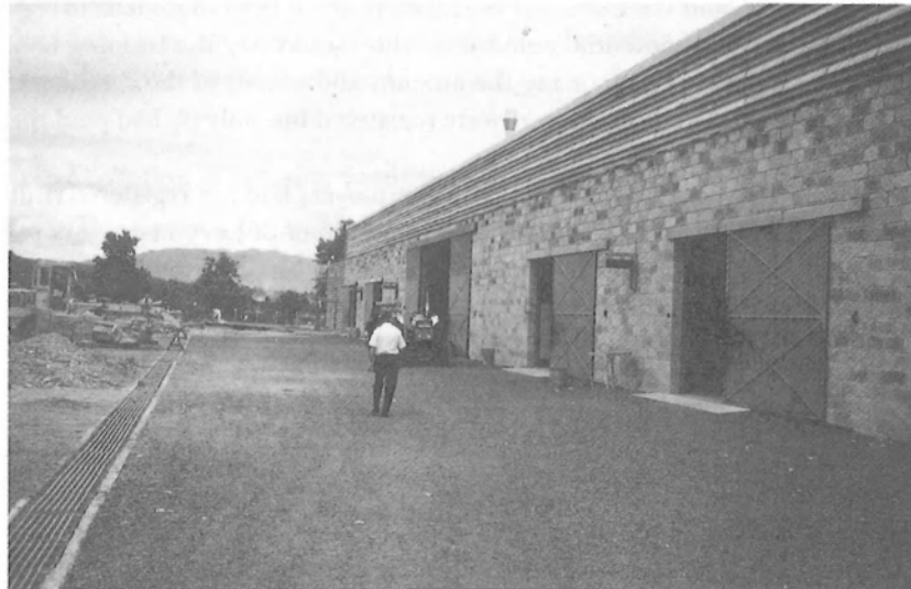
One of three Industrial Training Centres.
