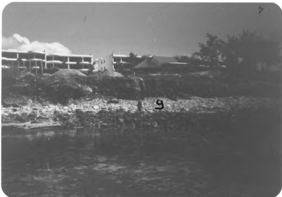
Plate 45 shows gravels (g) along Shanzu as an attempt to nourish the beach (September, 1990; Photo by J. Abuodha).
