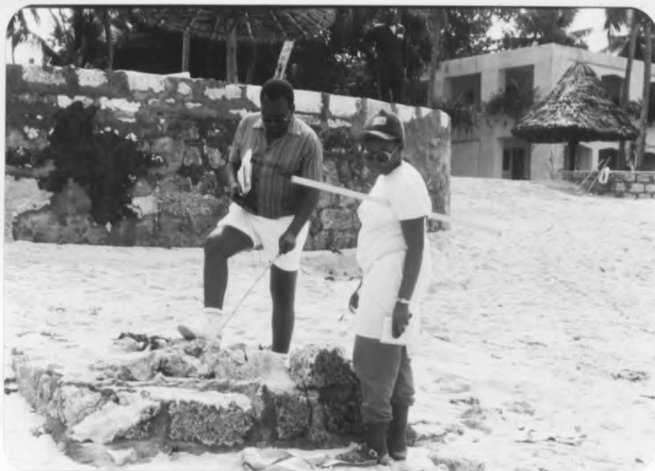
Plate 50 shows remnants of former seawall left 22 m seawards of the present wall at Likoni (June, 1991; Photo by S. Langat).
