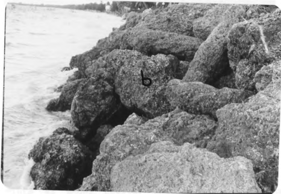
Plate 41 shows coastal protection using limestone boulders (b) along Bamburi (June, 1991; Photo by S. Langat).
