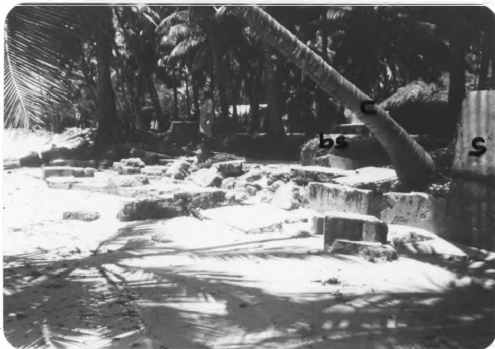
Plate 5 shows a 1 m beach scarp (bs), slanting coconut tree (c) and remnants of a seawall (s) at Kanamai as the results of wave action during a flood tide (September, 1990; Photo by J. Abuodha).
