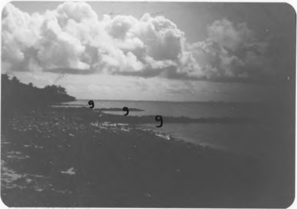
Plate 42 shows coastal protection using groynes (g) along Shanzu (September, 1990; Photo by P. Abuodha).
