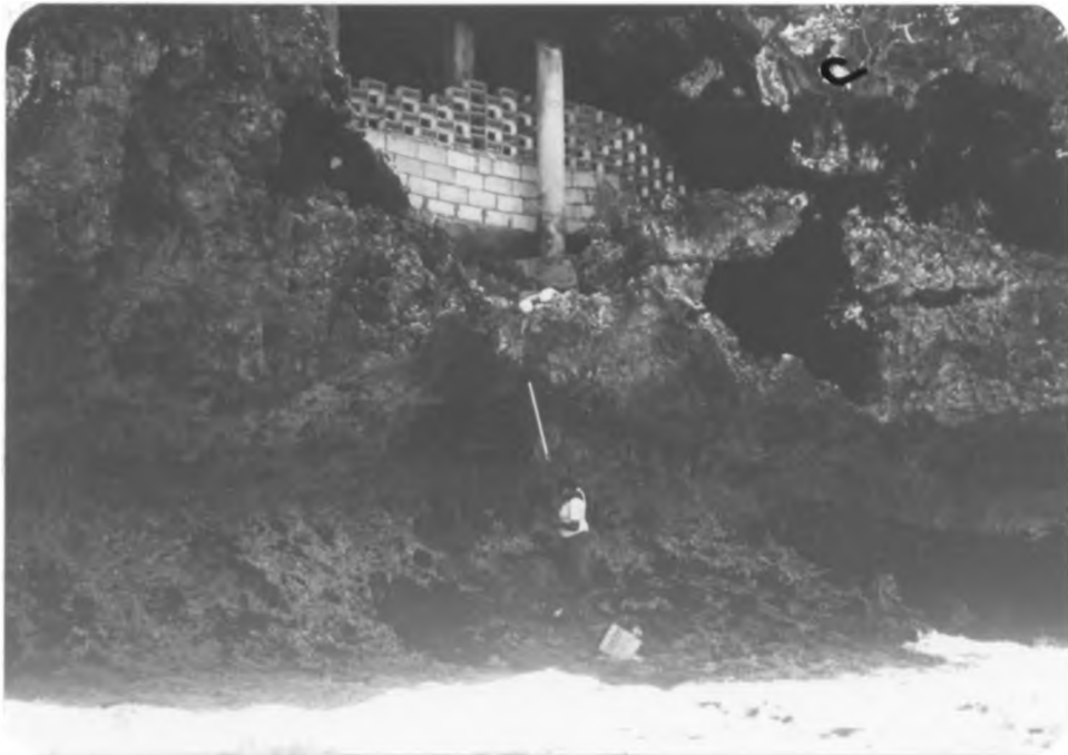
Plate 24 shows reinforcement of a hanging cliff (c) at Nyali. (September, 1990; Photo by J. Abuodha).
