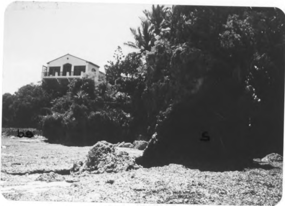
Plate 32 shows property on a cliff. Note stack (s) on the right and a beach scarp (bs) on the left of the plate at Nyali (September, 1990; Photo by P. Abuodha).
