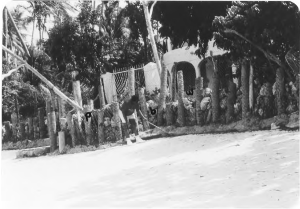
Plate 44 shows poles (p), limestone boulders (b) and wiremesh (w) at Kikambala being used for coastal protection (June, 1991; Photo by S. Langat).
