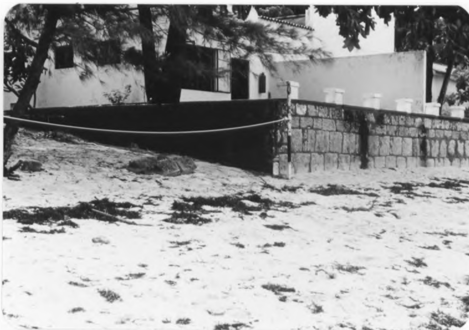
Plate 51 shows a recent seawall and a wall-in-the-making at Likoni. Note increased erosion at the end of the wall (June, 1991; Photo by S. Langat).
