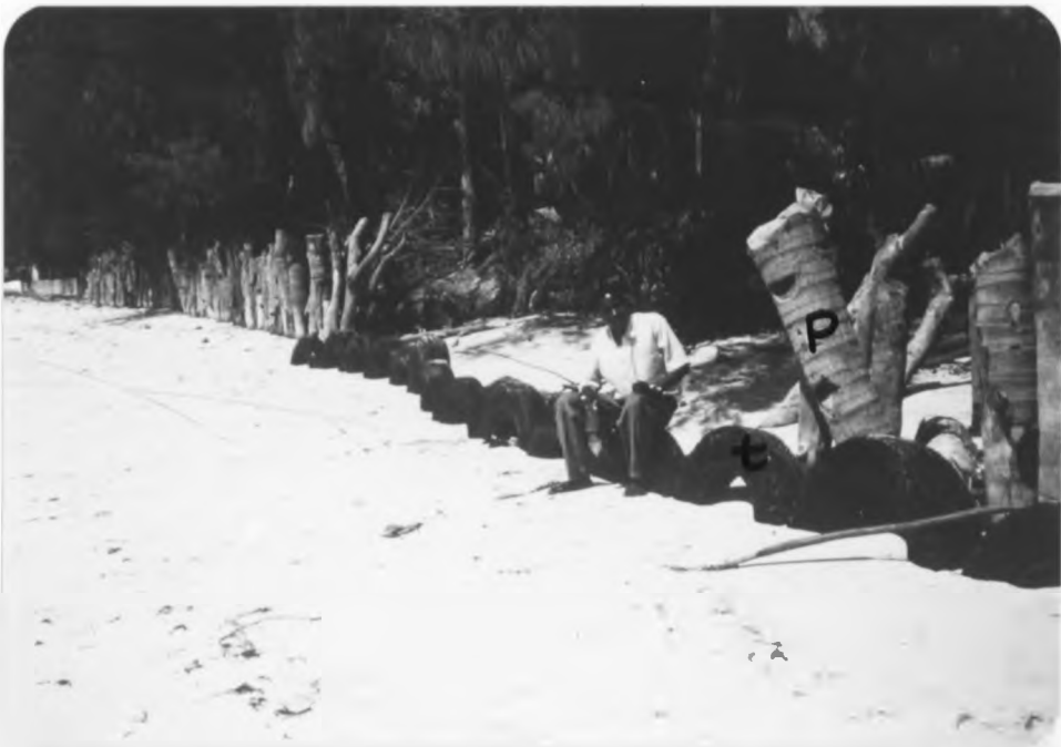
Plate 43 shows coastal protection using coconut poles (p) and used tyres (t) at Kikambala (September, 1990; Photo by P. Abuodha).
