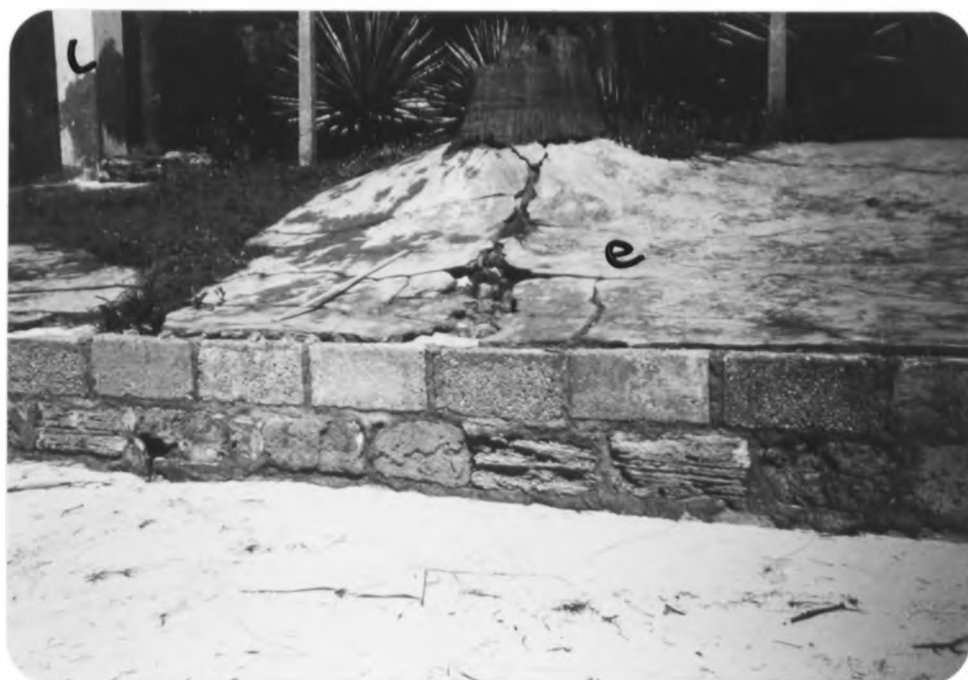
Plate 53 shows an embarkment (e) at Kikambala. Note level (l) of splash water mark on the left of the plate on a gate frame (September, 1990; Photo by P. Abuodha).
