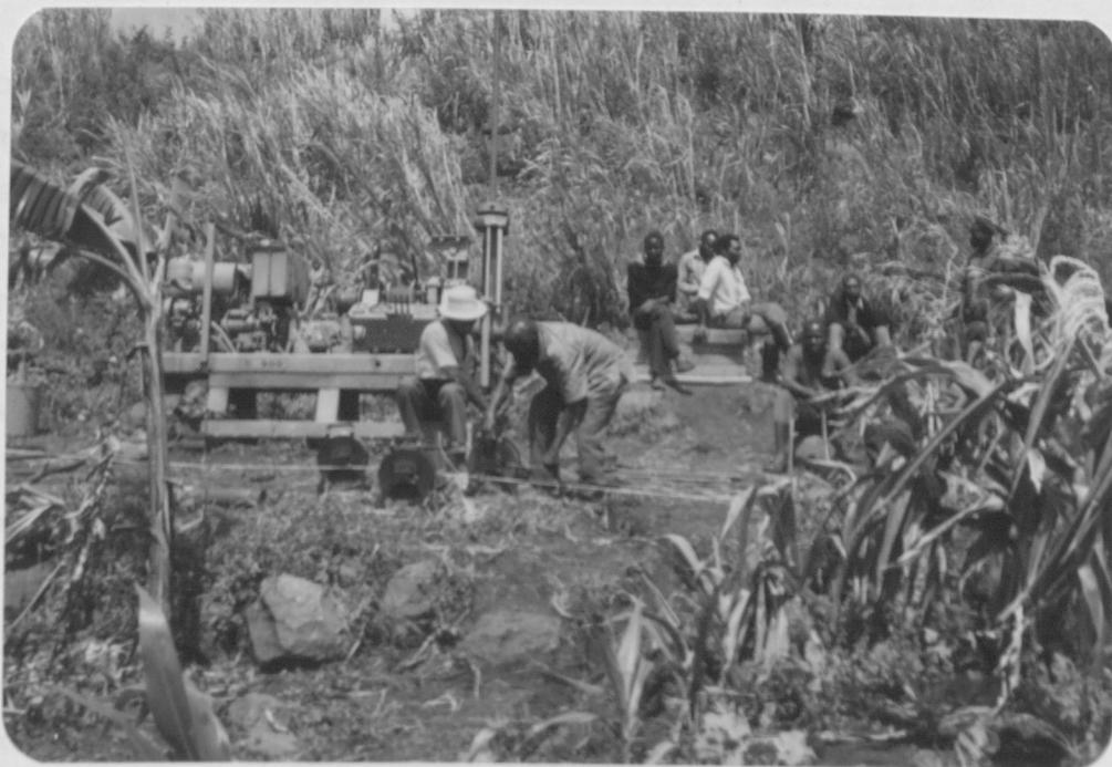
Plate 4.4 Core drilling in progress at BH2. Note V.E.S. S17 being conducted next to the borehole. The spread is along the flat valley bottom with the steep rise on the right abutment seen on the background.
