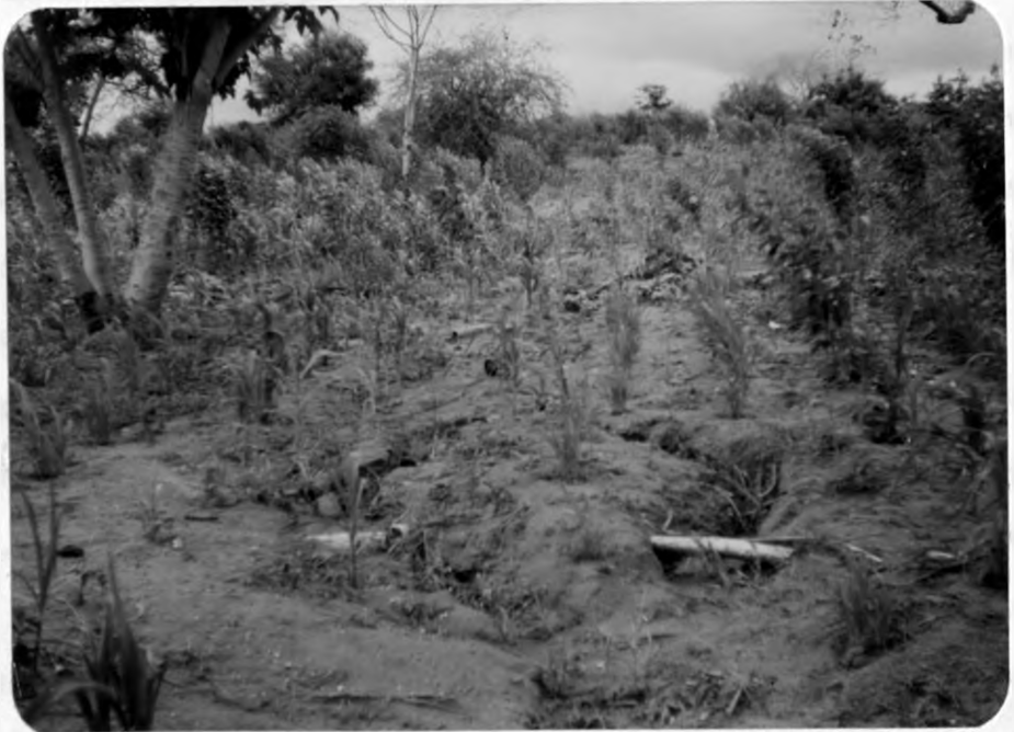
Plate 25. Rill erosion on a gentle slope. Lack of ground cover paved the way to rill erosion (Photo taken in April 1989).
