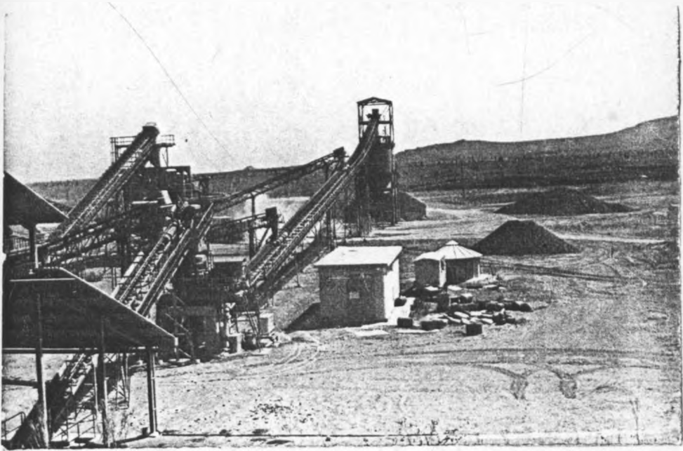
PLATE NO. 22: Part of the advanced technology used at the quarries. Similar efforts are needed in rehabilitation programmes.
