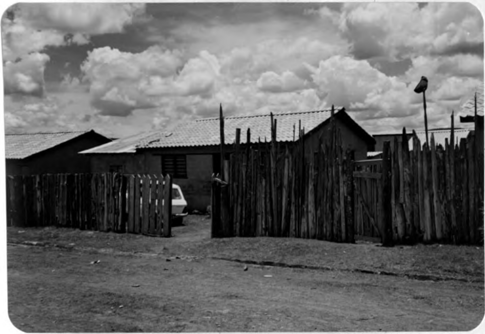
PLATE 4.5; NYAHURURU TENANT PURCHASE HOUSING SCHEME.
