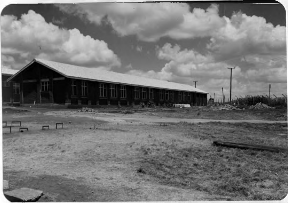
PLATE 3.5: KANGEMI, NAIROBI Block of classrooms at St. Joseph The Worker Primary School.
