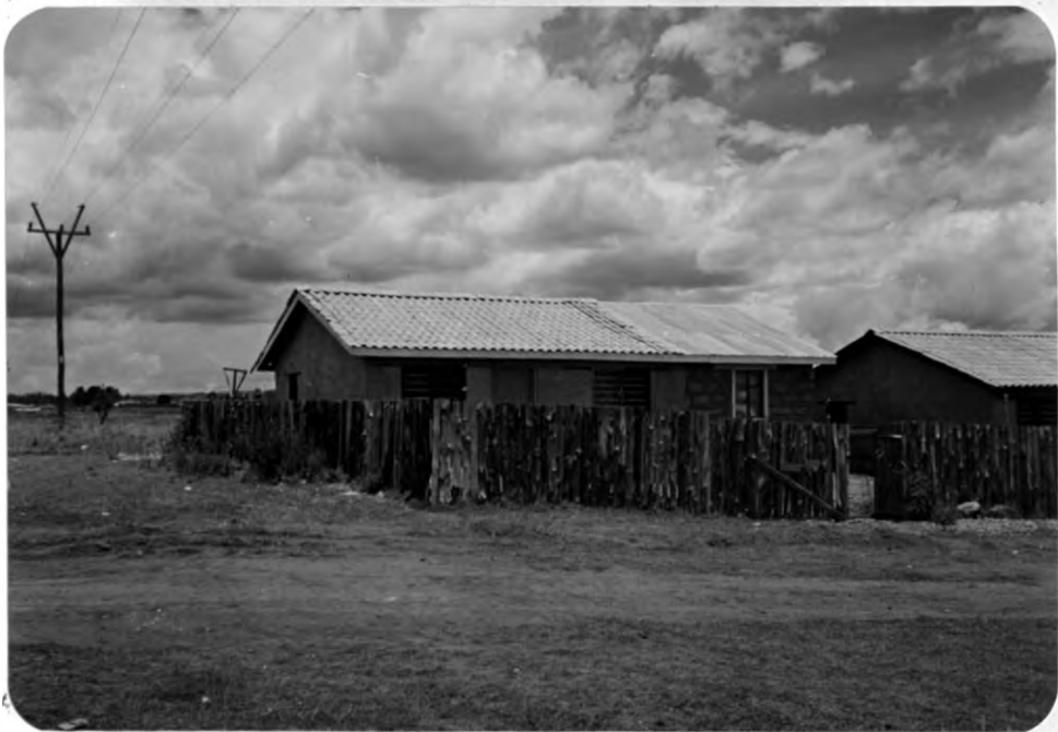
PLATE 4.6; NYAHURURU TENANT PURCHASE HOUSING SCHEME.
