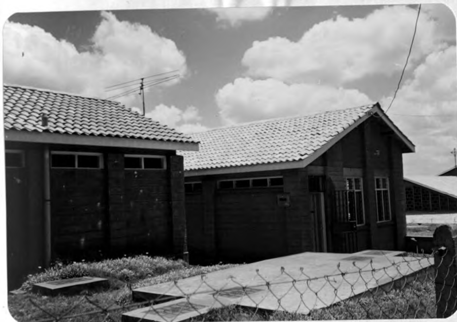
PLATE 4.11: KANGEMI, NAIROBI St. Joseph the Worker Parish, Kangemi, Nairobi. Offices and Residence built of FCR tiles and soil blocks still in very good condition.
