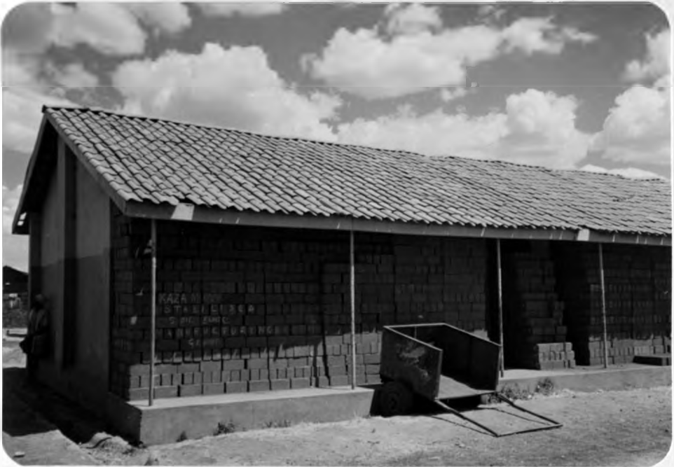
PLATE 3.10: KOROGOCHO, NAIROBI Completed classroom at Korogocho Primary School. Note the stabilized soil blocks stacked on the verandah for future use.
