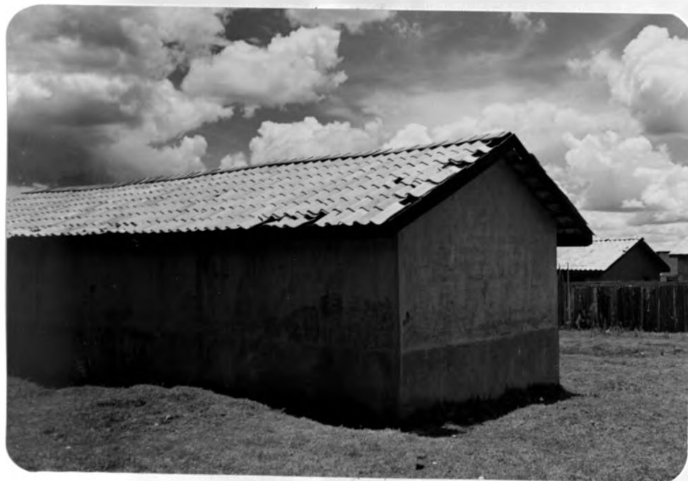
PLATE 4.1; NYAHURURU TENANT PURCHASE HOUSING SCHEME.
