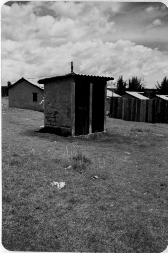
PLATE 4.7; NYAHURURU TENANT PURCHASE HOUSING SCHEME.
