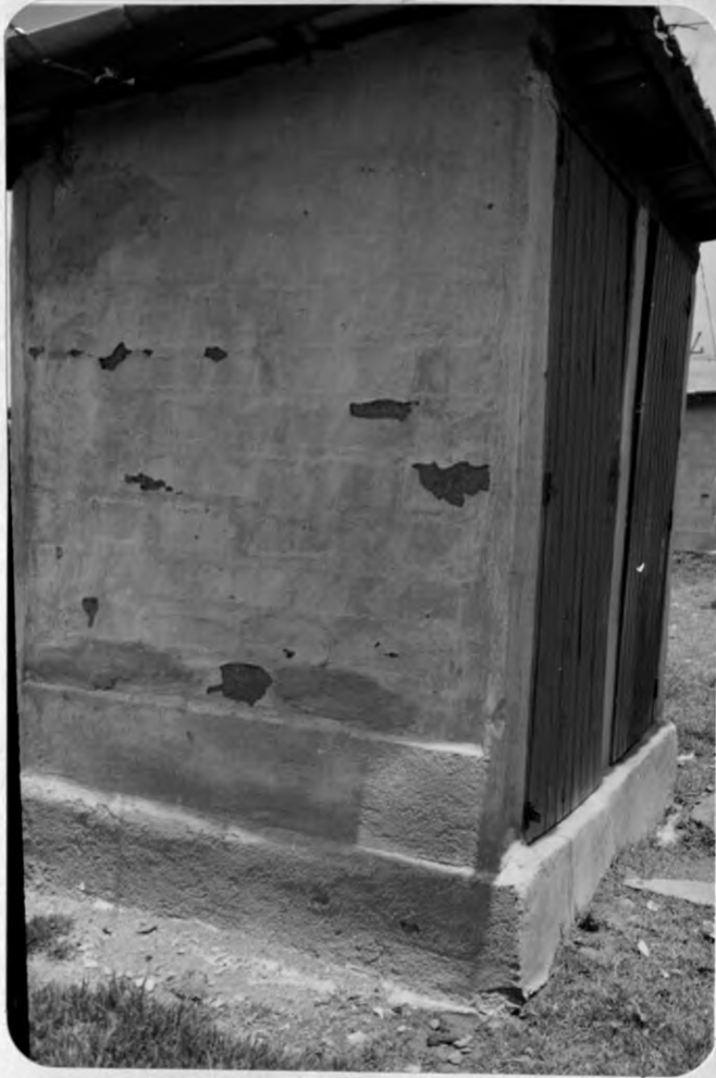
PLATE 4.8; NYAHURURU TENANT PURCHASE HOUSING SCHEME.
