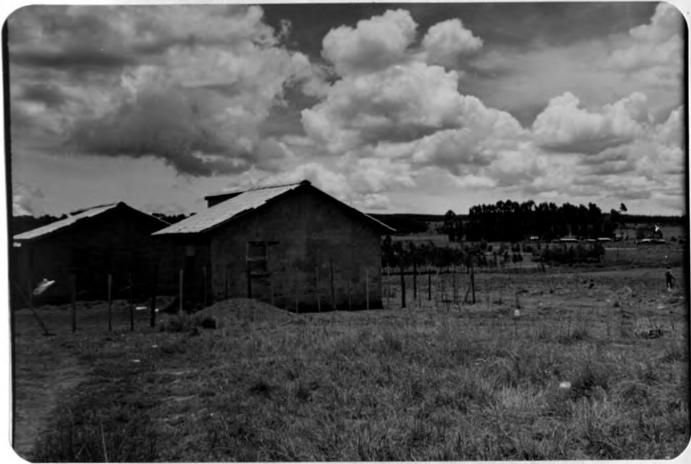
PLATE 4.2: NYAHURURU TENANT PURCHASE HOUSING SCHEME.
