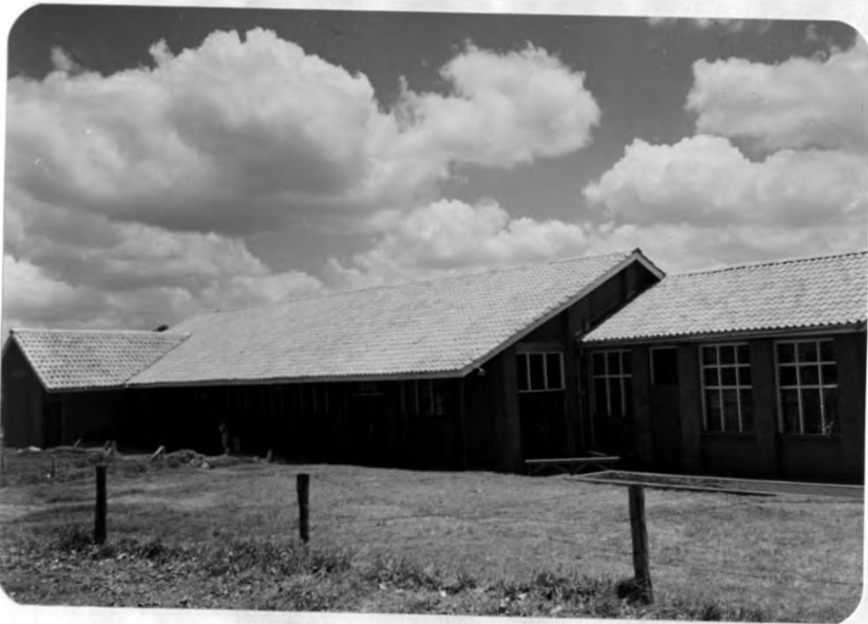
PLATE 3.6: KANGEMI, NAIROBI Block of classrooms at St. Joseph The Worker Primary School.
