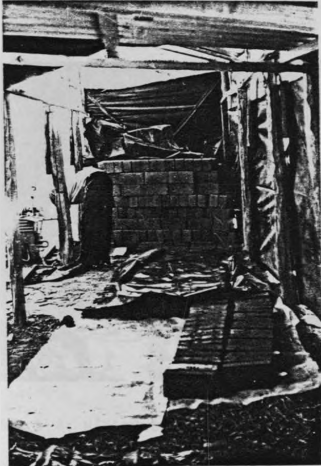
PLATE 3.7: CURING OF SOIL-CEMENT BLOCKS
