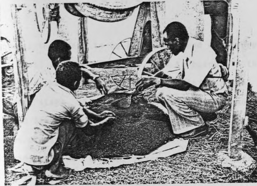
PLATE 3.5: MIXING OF SOIL AND CEMENT
