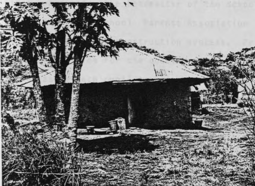
PLATE 3.2: TEACHERS' HOUSE AT LAMBWE PRIMARY SCHOOL
