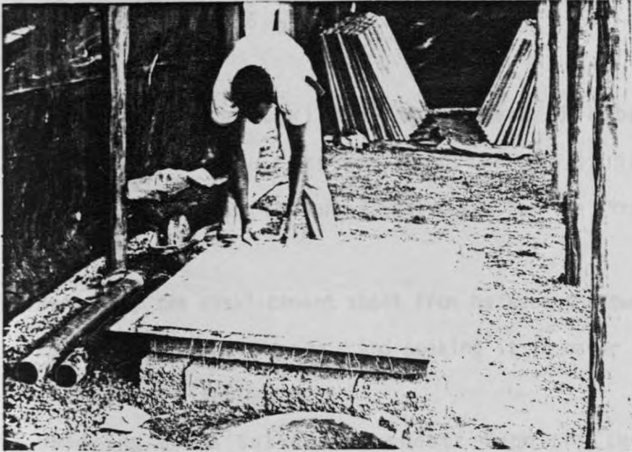
PLATE 3.9: PREPARING A FLAT SISAL-CEMENT SHEET
