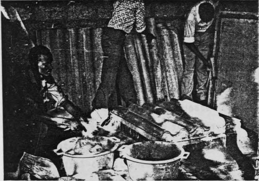
PLATE 3.8: MIXING OF CEMENT, SAND, AND CHOPPED SISAL
