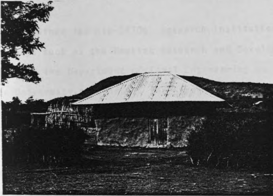
PLATE 3.3: TEACHERS' HOUSE AT NYAMUGA PRIMARY SCHOOL
