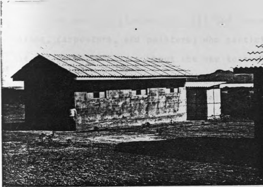
PLATE 4.4: IMPROVED TEACHERS' HOUSE AT NYAMUGA PRIMARY SCHOOL
