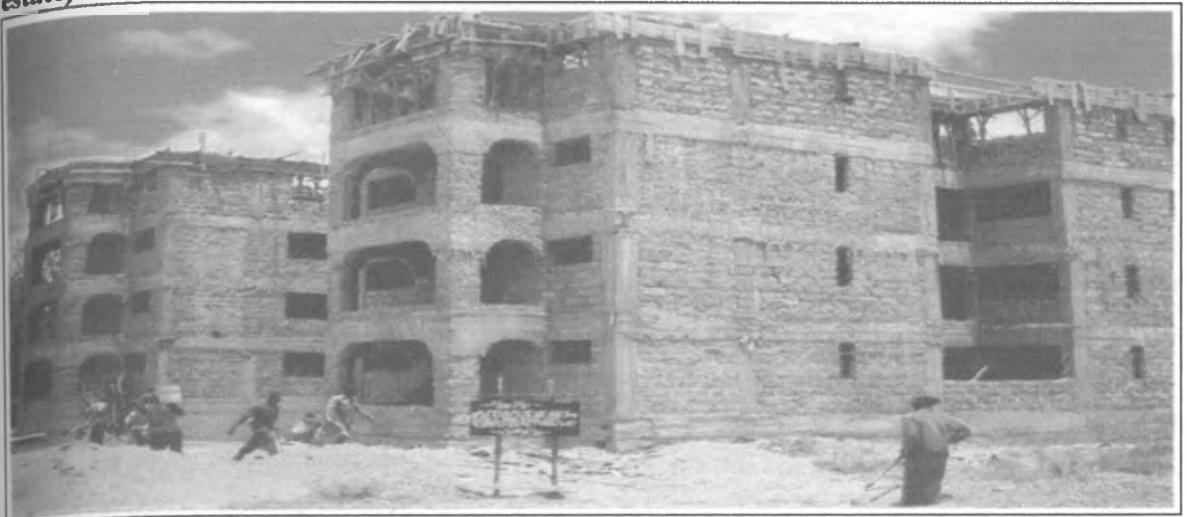
Plate 4: Multiple dwelling units under construction within a low-density zone(Senior Staff estate).
