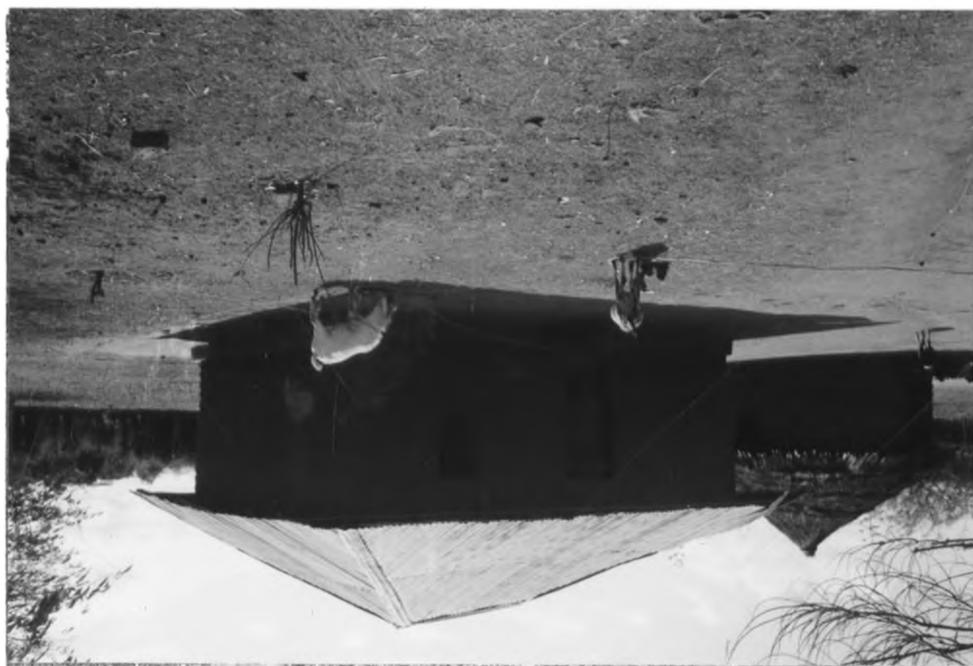
Plate 4.2: Rectangular house made of mud brick walls and a corrugated iron sheet roof.
