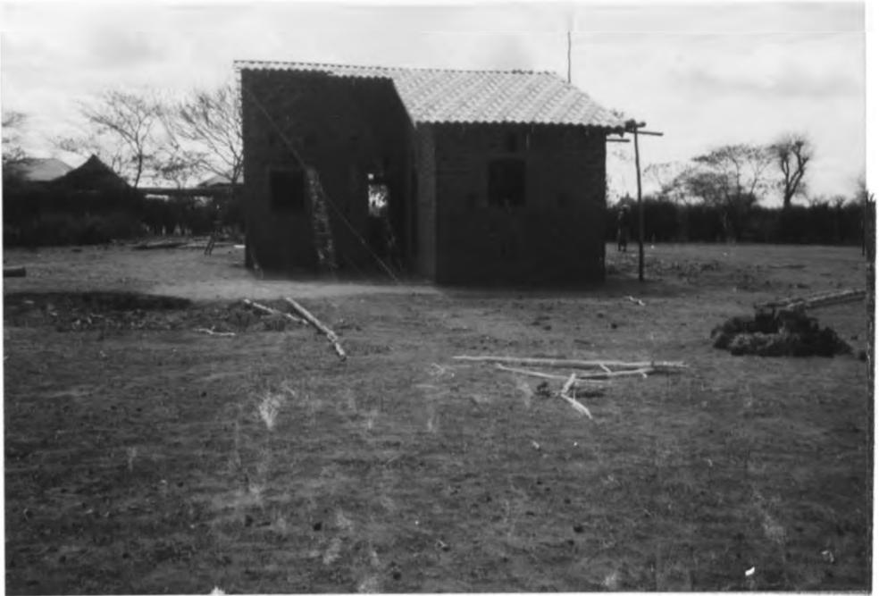
Plate 4.5: House constructed with concrete block/natural stone walls and a tile roof. These designs are mainly constructed by the Kauwi Muugano project
