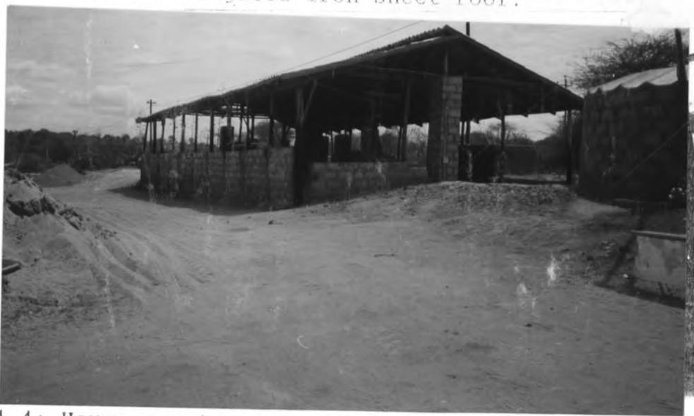
Plate 4.4: House constructed with concrete block walls and a corrugated iron sheet roof
