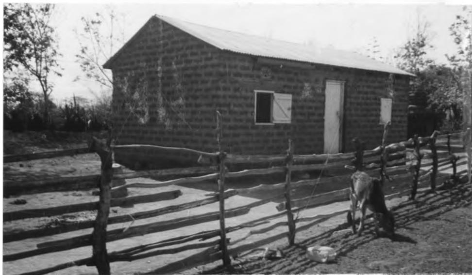
Plate 4.3: Rectangular house made of fired brick walls and a corrugated iron sheet roof.
