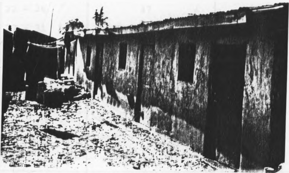
Plate 3: A mud plastered house in Kawangware.
