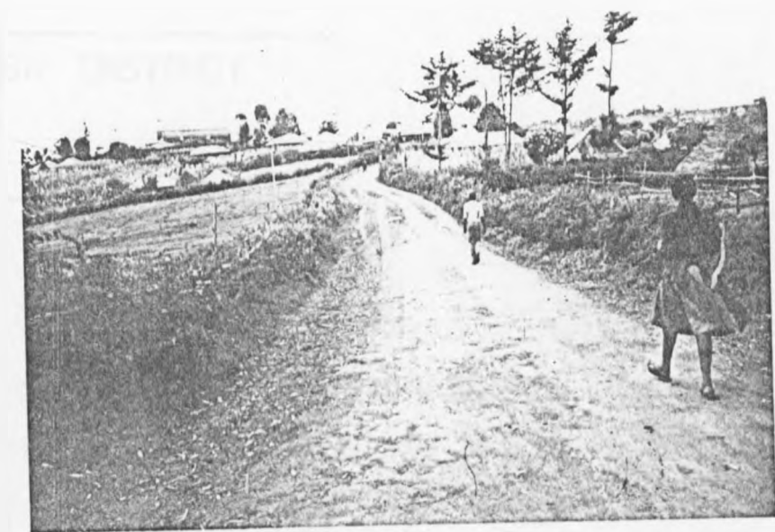
Plate No, 9 : Tarmaced section of the road to the factory.
