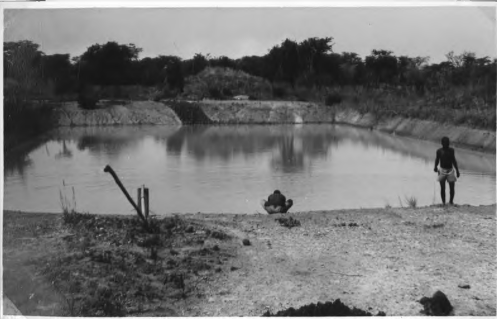
BUNYORO : One of a series of 750,000 gallon valley tanks being built with the assistance of the Federal German Government. Tanks are rapidly replacing dams as the main form of artificial water supplies for cattle in Uganda. The tank shown above is situated on the Bunyoro Growers' Cooperative ranch.
