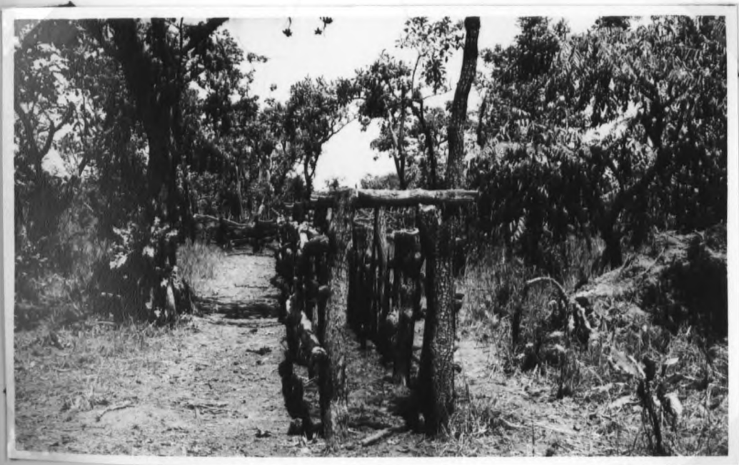
ACHOLI: A 'crush' built for inspecting and treating animals in transit from the county markets of south-eastern Acholi. Animals are driven through slowly to be inspected and innolculated in order that disease may not be spread by trade movements.
