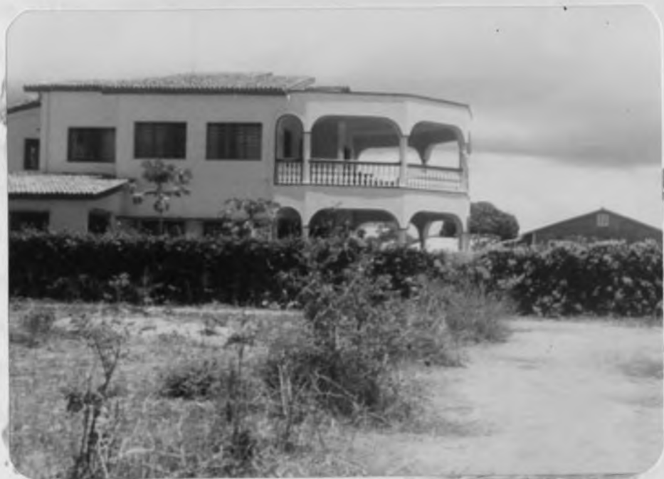
Plate 10: Example of one of the modern houses coming up at the outskirts of Malindi old town.
