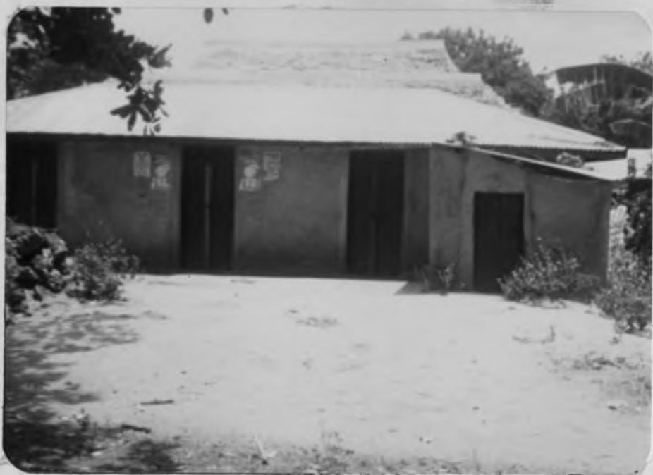
Plate 5.: A "long store" in Kaloleni, built of concrete blocks and G.C.I. On the right is the toilet.
