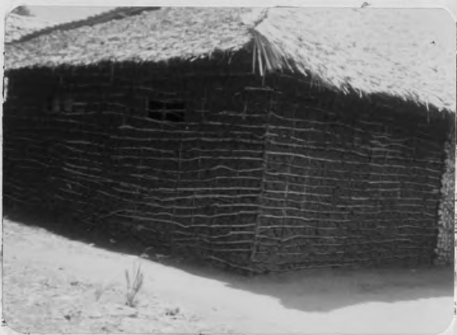
Plate 2: A completed mud and wattle house with Makuti roof in Majengo, Malindi. At the back is the courtyard and utility rooms.
