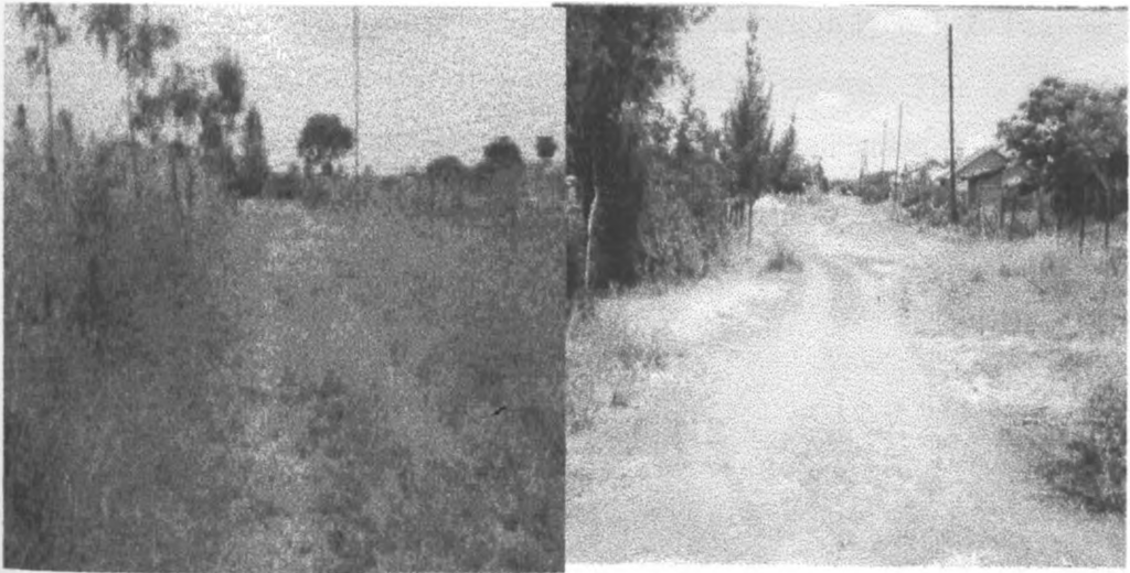
Plate 5- 2: Poor maintained roads.
