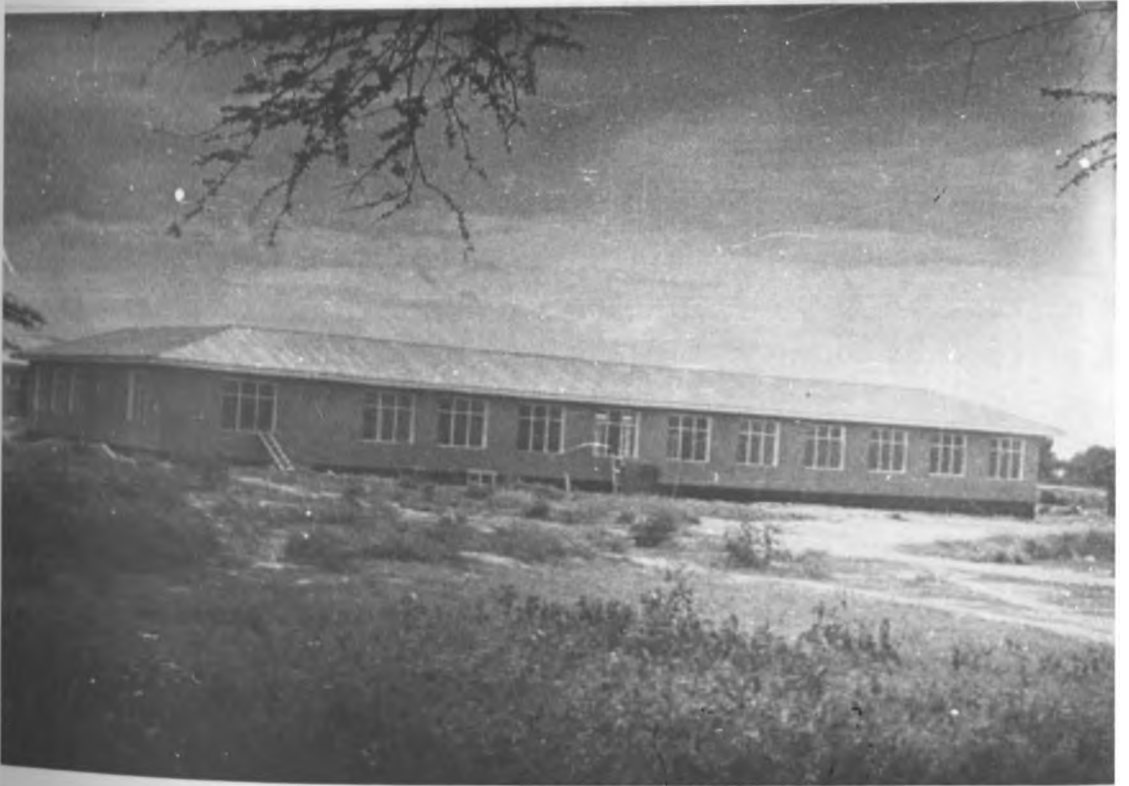
Plate 4. Temporary Offices for Government Technical Divisions
