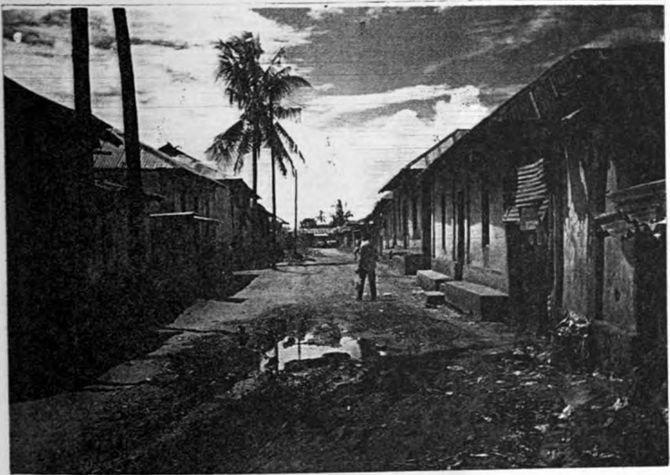
Plate 2. Part of the planned swahili settlement at Kongowea. Some services were provided (water,electricity and access roads). Note the kiosks coming up in the neighbourhood and poorly maintained houses becoming almost inhabitable.
