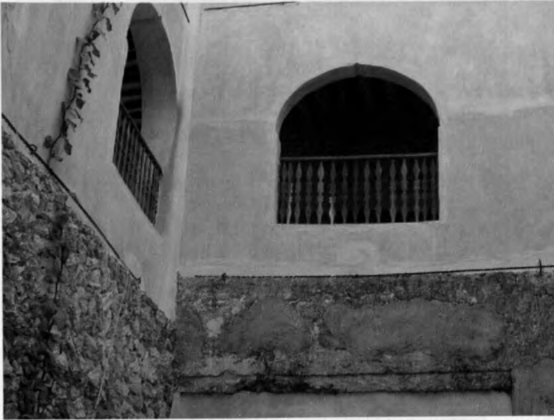
Plate 6:6 Restored Lamu pointed arch 158
