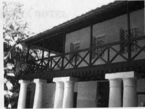
Mombasa Serena Twin column support system
