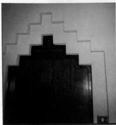
Plate 4:8, Nairobi Serena hotel, stepped door arch on main doors
