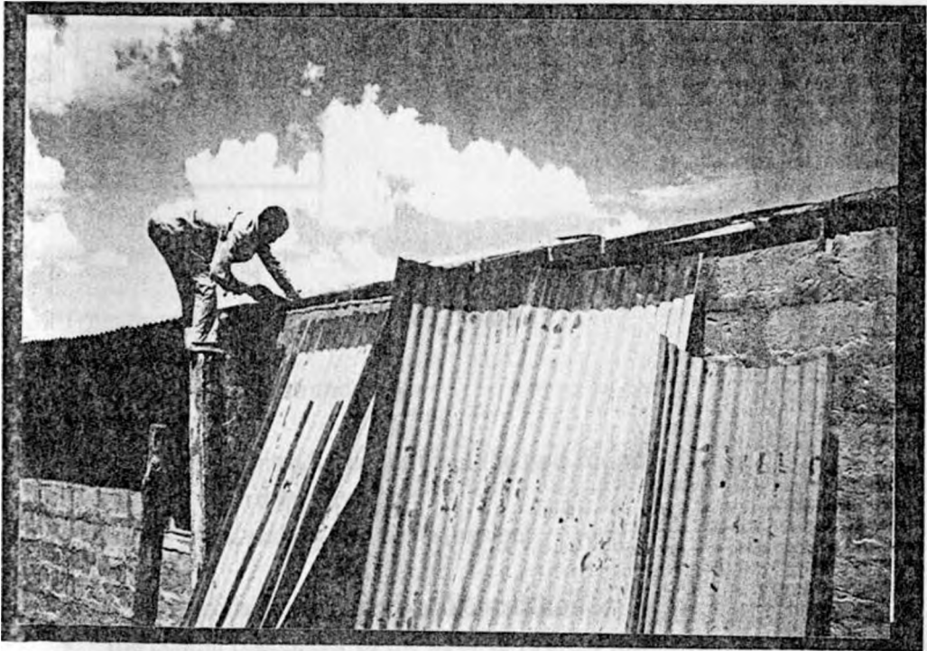
Photo 4.11 Transformation; removal of original GCI for elevating roof
