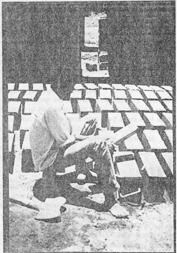
Photo 2.4 Block making by local 'fundi' at Bung'oma TP scheme
