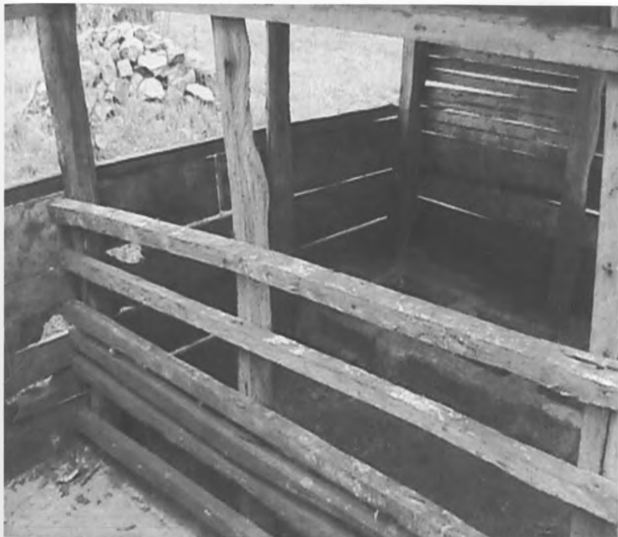
Plate 4.2: A model pig house constructed by a researcher in Homa Bay District 2010.
