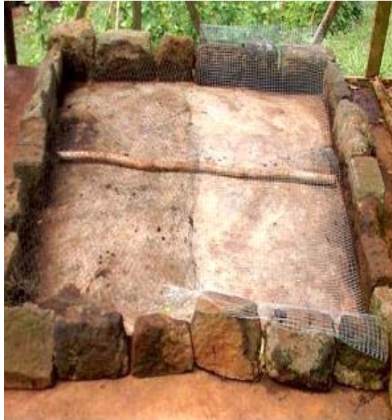
Figure 4. A vermicomposting bed with rock walls and concrete floor (Step 1).
