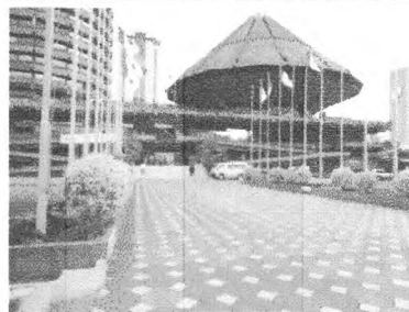
K.I.C.C paving blocks ground surface. Consistent use of the paving materials and pattern developed a decorative rhythm.
