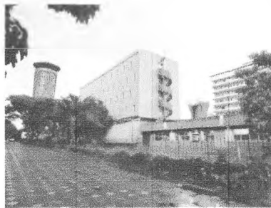
The gates and fences restricted movement and controlled security.
