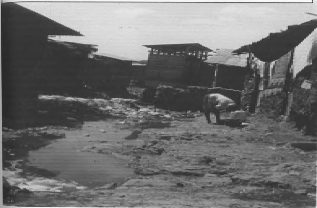
Plate 6.2: Depicts Stagnant Water next to Residential Houses in Kibera Division
