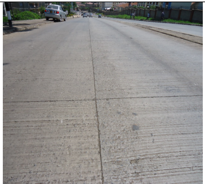
Typical longitudinal joint
