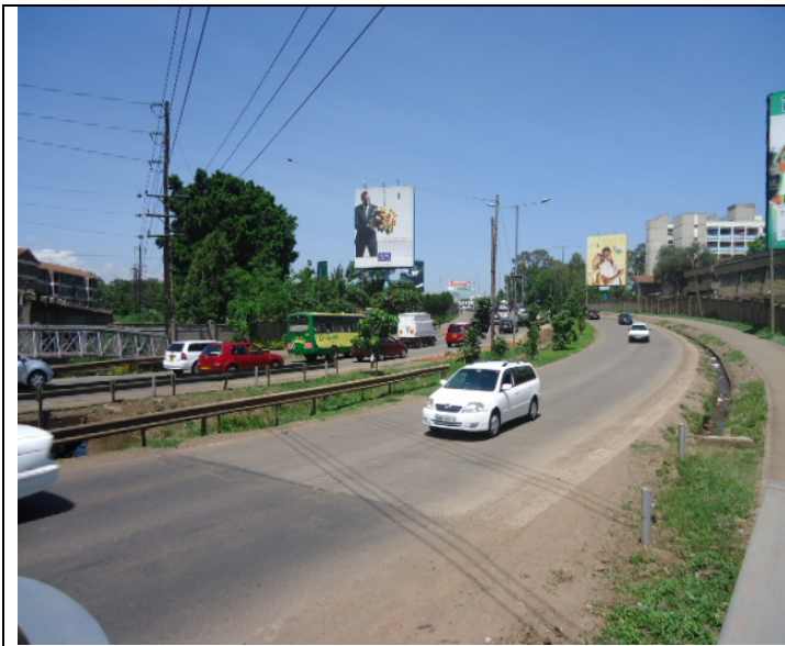
Concrete pavement at Mbagathi Way, Kenya
