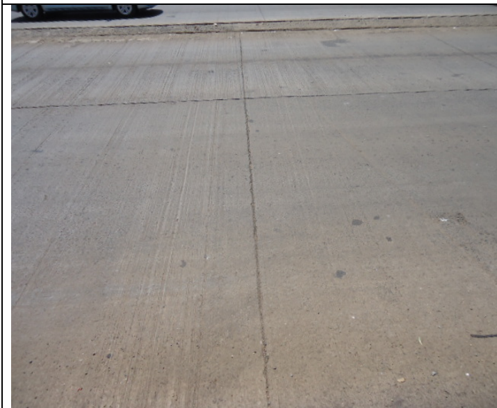
Typical tranverse joint on the road
