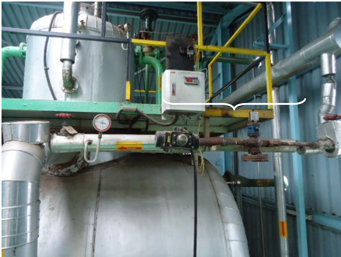
Figure 2-7: Deaerator steam injection system
