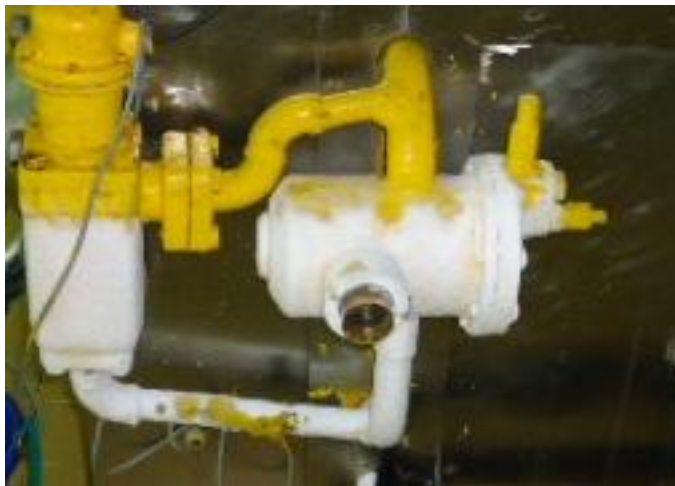
Figure 4-25: Unlagged Sections.
